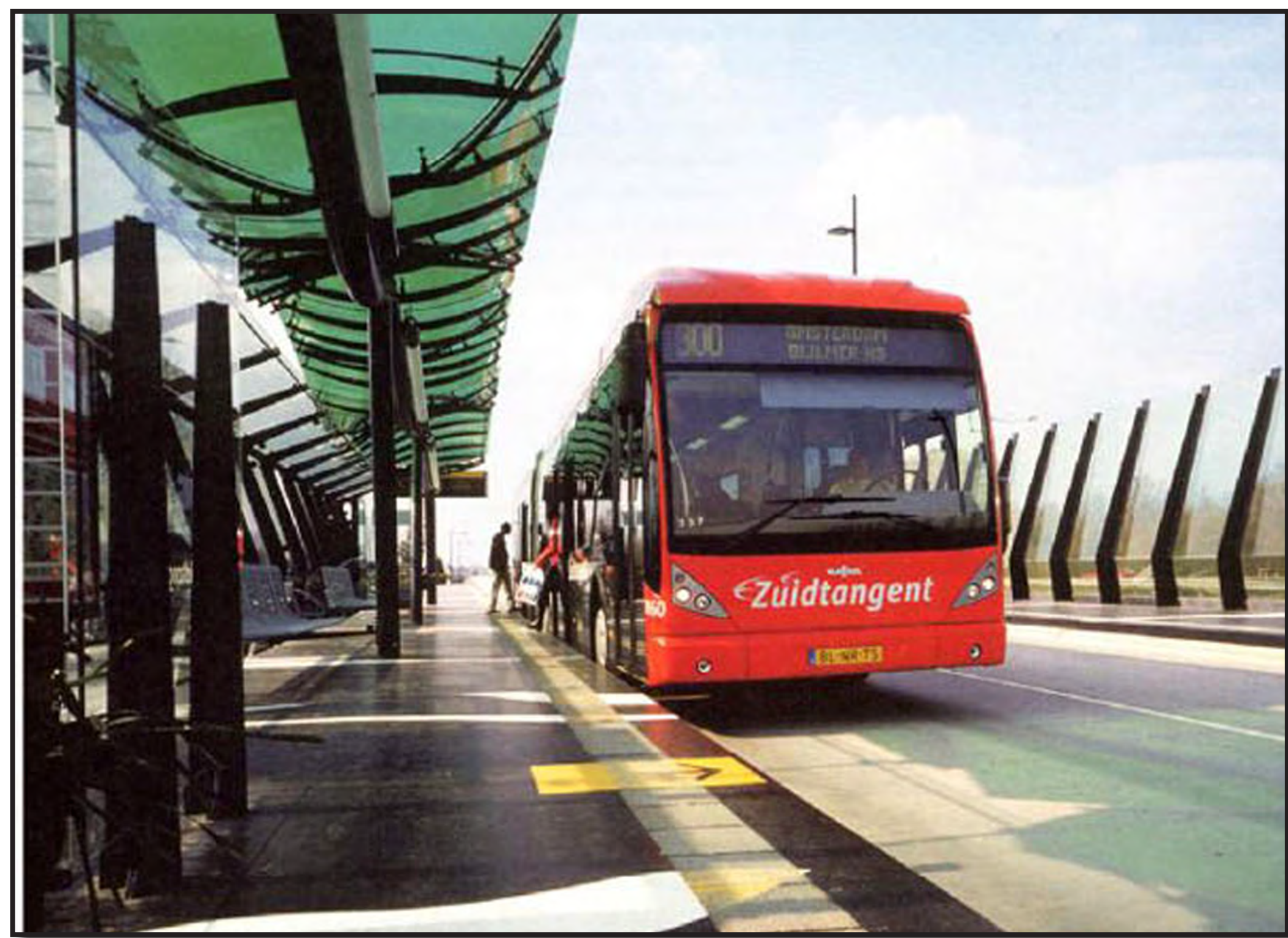
BRT Station - Schiphol, Netherlands
